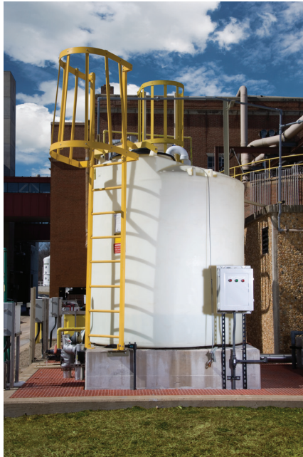
To extend longevity, you can store corrosive oxidizing chemicals in an XLPE tank with an antioxidant barrier system.
